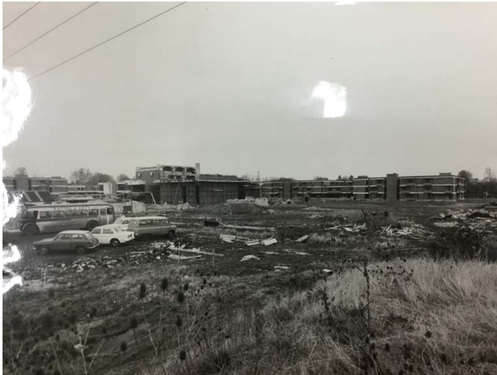
The building site c. 1964 (CCPH/5/2) © Lafayette Photography
